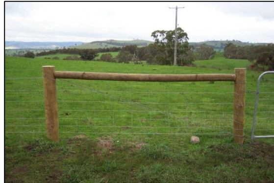
Figure 2: Ring lock or hinge joint and box type stay.
