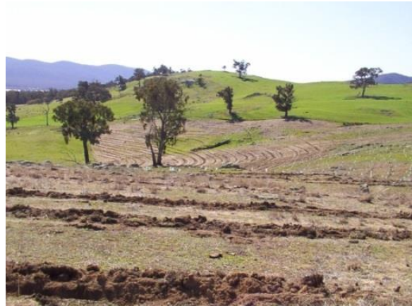
Figure 18: Blanket sprayed and seeded.
