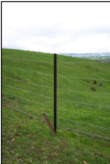
Figure 3: Undulations in fence require pegging down to reduce pop outs.
