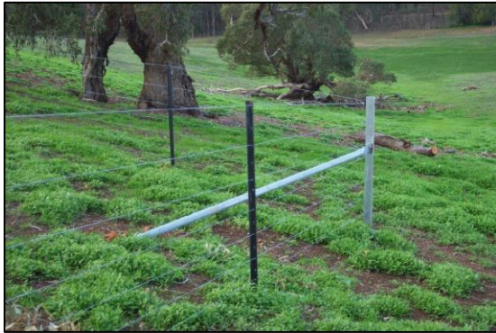
Figure 1: Plain wire fence with diagonal stay.
