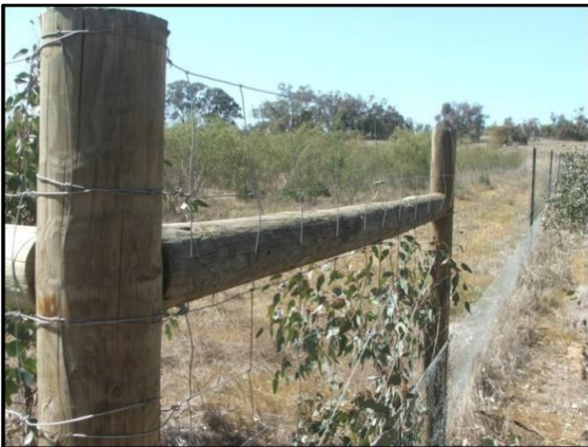
Figure 5: Kangaroo proof Ring lock/ hinge joint 2m fence with rabbit netting to 900mm.
