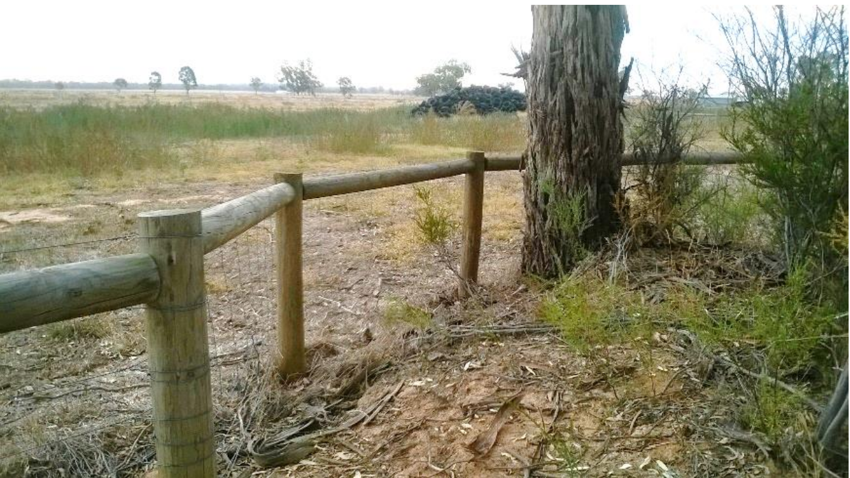
Figure 6: When existing trees are along a fence line fence around the tree inside the property boundary.
